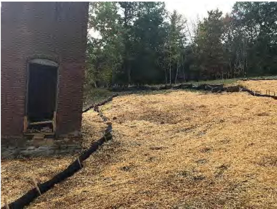
Fig 12: Swale upslope of the cable house at the Eversource property/west side of the bay. Viewing southwest. (09-30-20)
