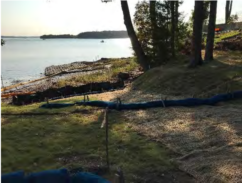
Fig 1: Jute matting securing sod on slope below manhole at Gundalow Landing/east side of the bay. Viewing west. (09-25-20)
